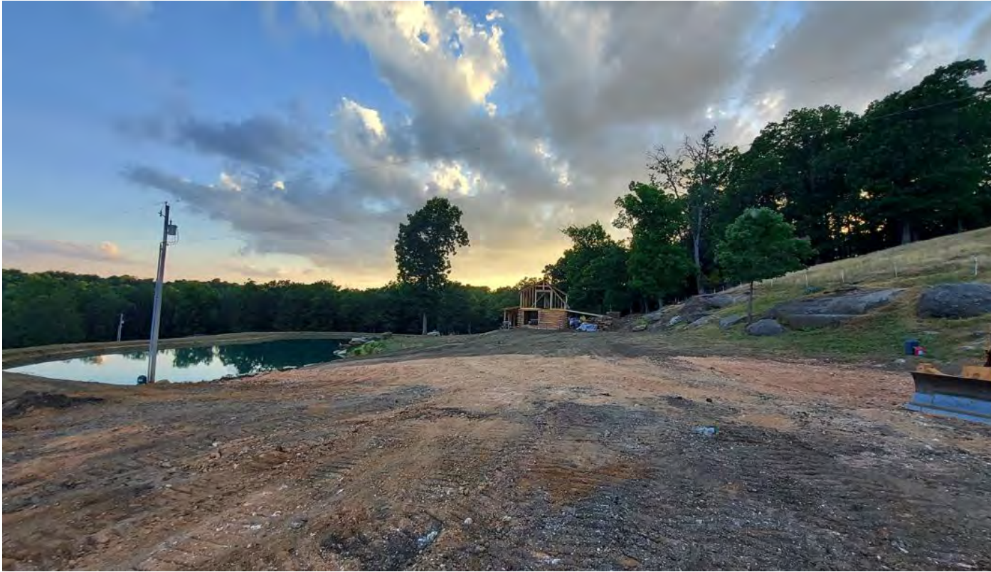
Facing S towards cabin
