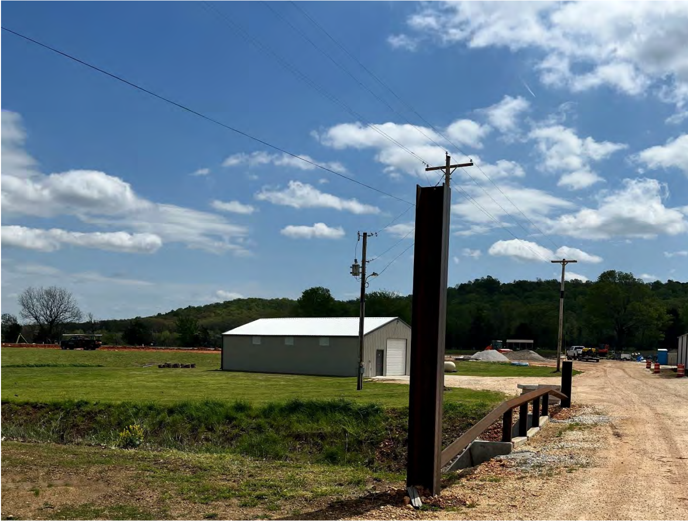
Facing east toward building in construction
