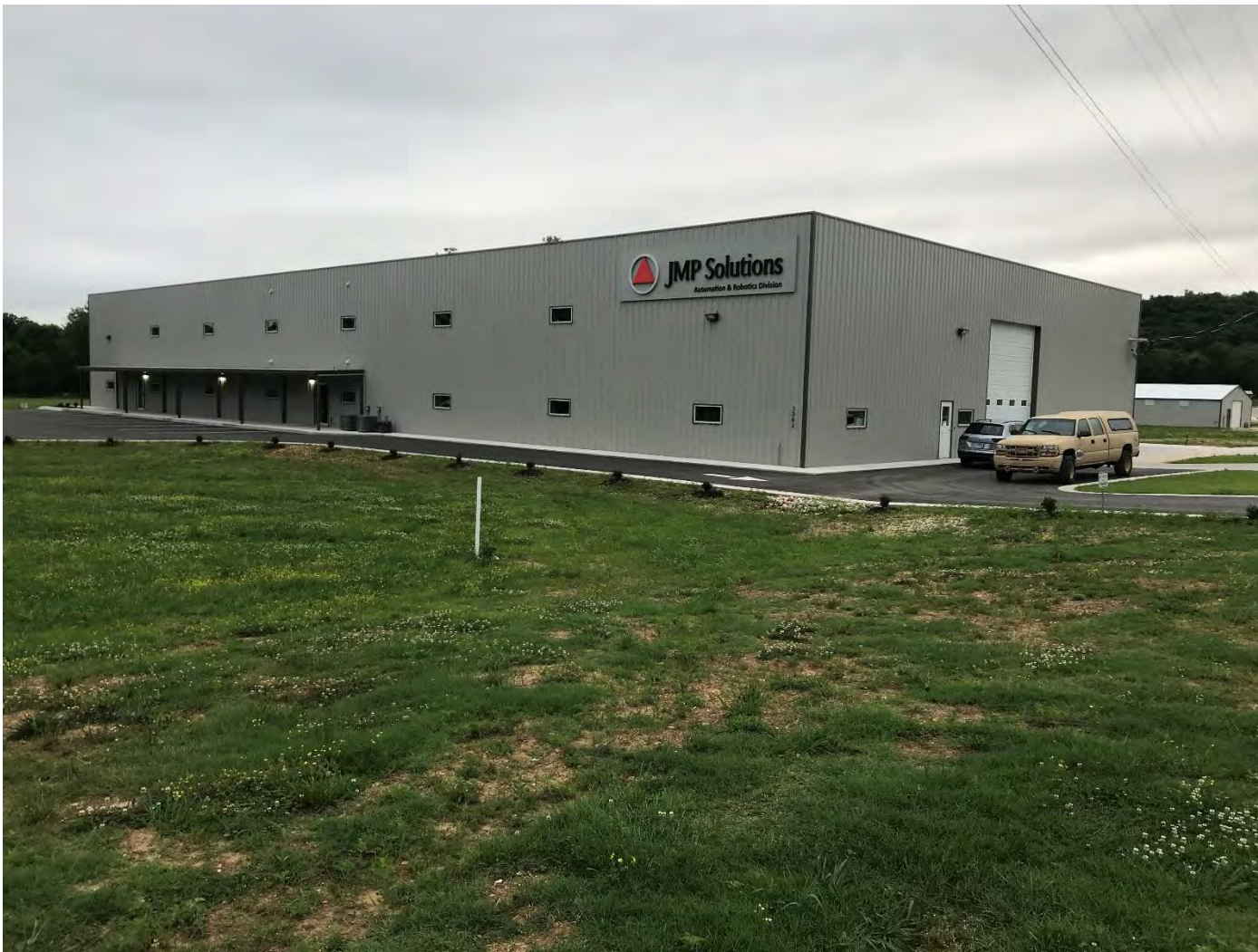
Facility on Cato Springs (in operation)
