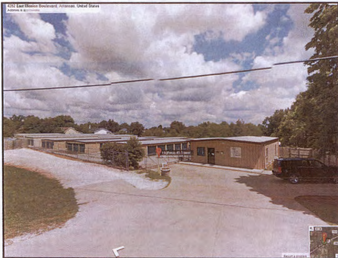
Figure 2. Tower Storage units. Photo from Google Earth.
