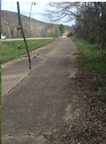
(existing portion of old Hwy 71 – possible Apron)
