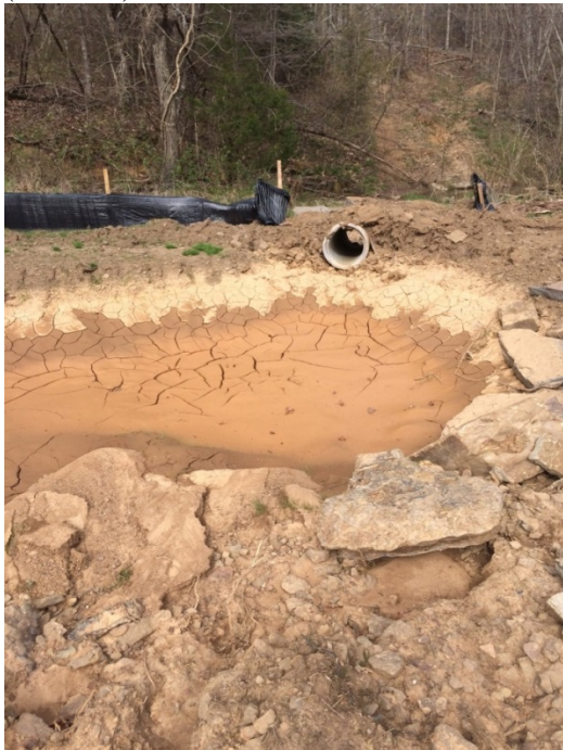
(existing sediment pond)
