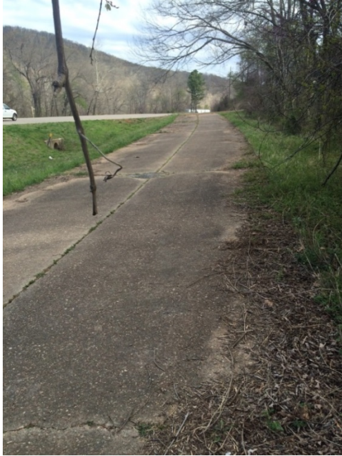
(Existing portion of old Hwy 71 – possible apron)
